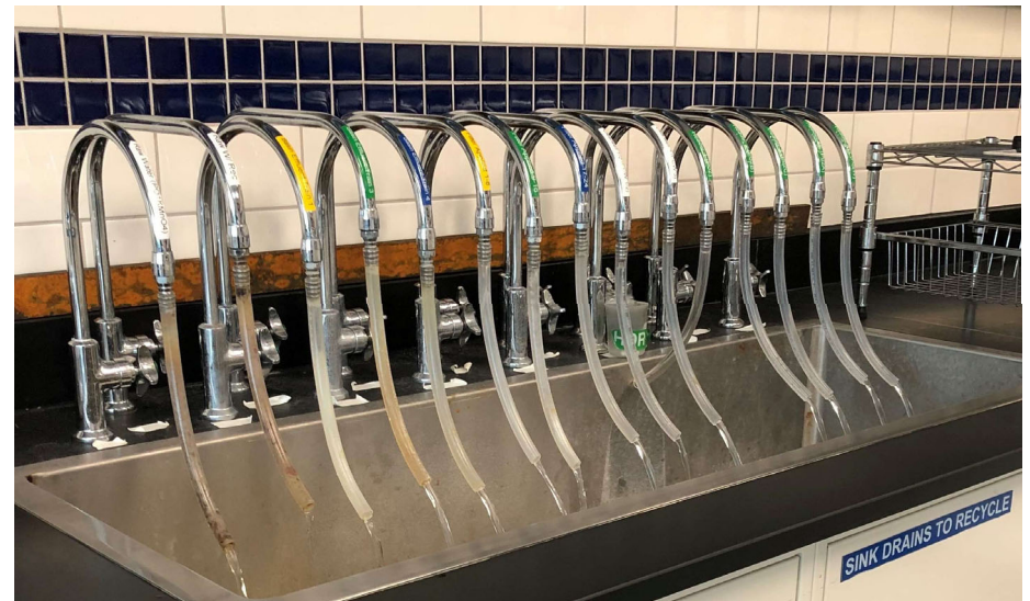
Corbalis Water Treatment Plant Sample Taps
